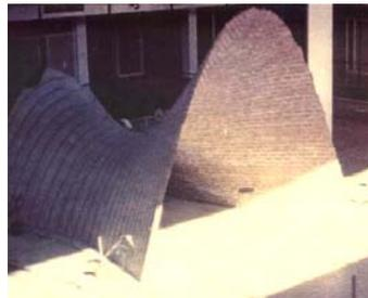
**Fig. 5** The straight-line generated masonry saddle vault constructed by Prof. V. Michelson's architecture students at the U. of Minnesota circa 1960s. Photo by Francis Bulbulian.
